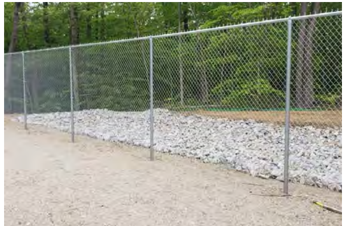
Swale installed beside compound
