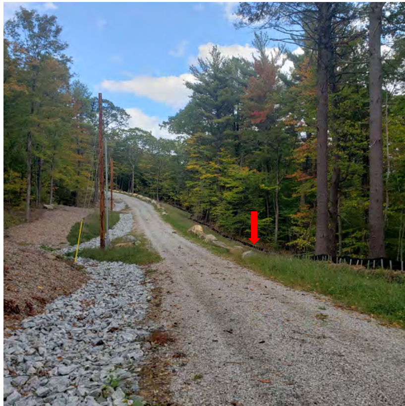
Monterey, MA – Perimeter Erosion Control until Final Stabilization
