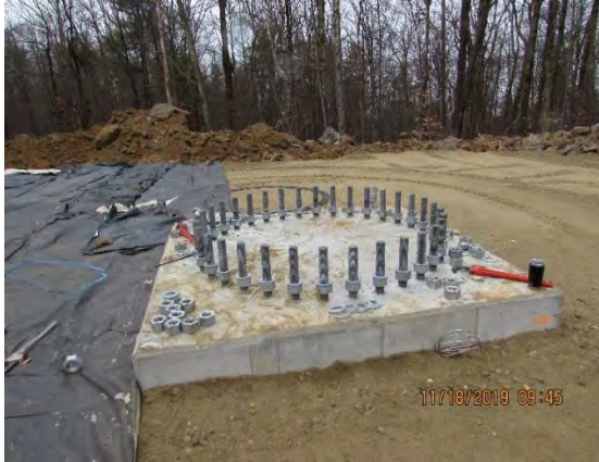
Tower foundation and bolts in place
