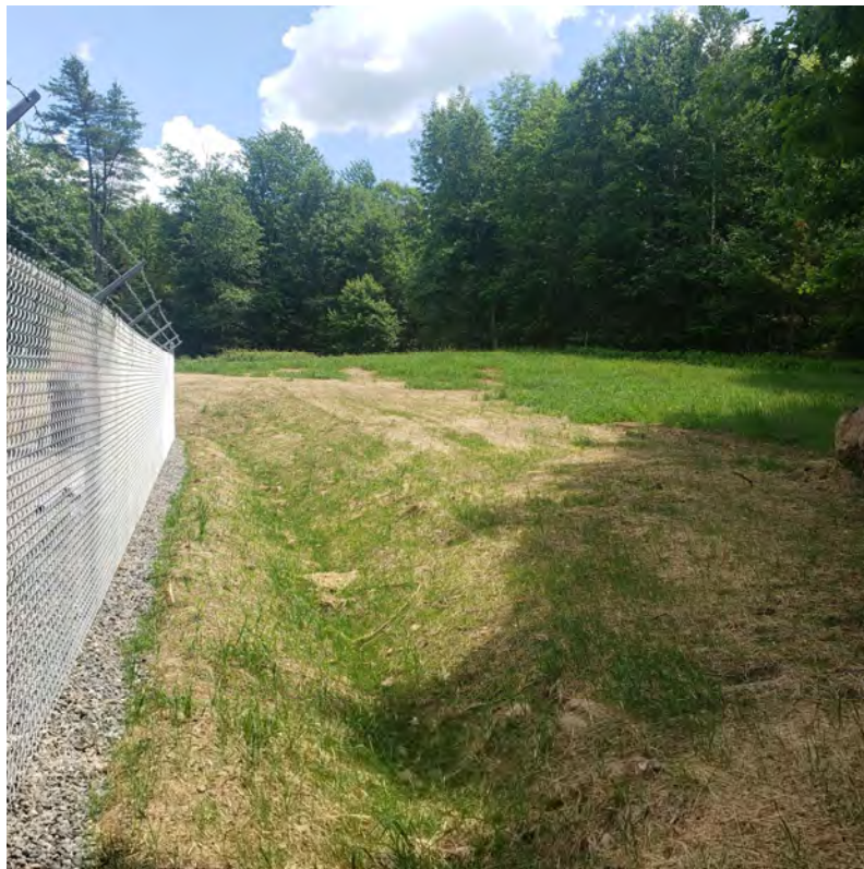
Bath, NH – Disturbed Areas with Mulch Stabilization until Vegetation Establishment
