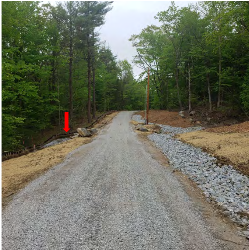
Monterey, MA – Disturbed Area Mulch Stabilization and Downhill Erosion Control
