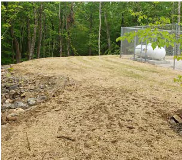
Disturbed areas seeded and hayed
