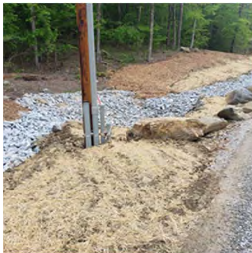
Plunge pool and underground conduit
