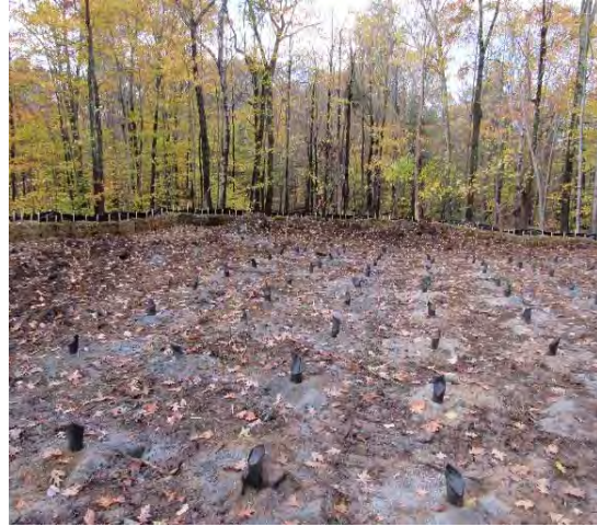
Blasting set up
