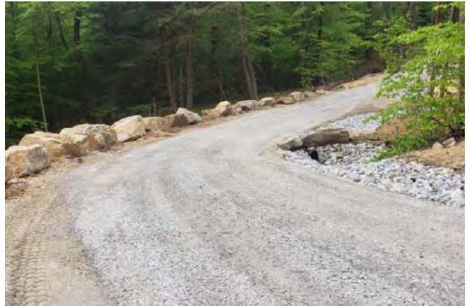
Access road, swales and boulders
