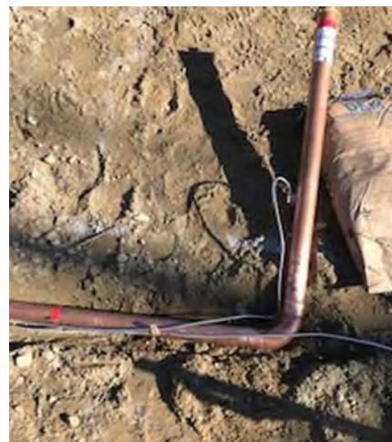
Electrolytic ground rod
