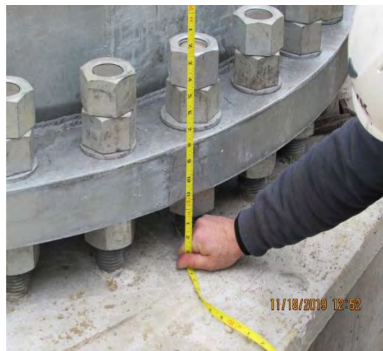
Tower base on anchor rods, bolts tightened
