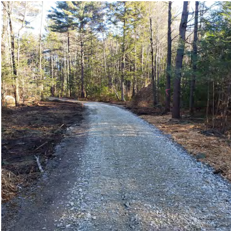
Henniker, NH – Wood Mulch Stabilization along Driveway
