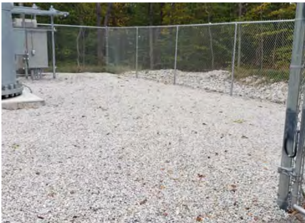
Stone Finishing placed within compound.
