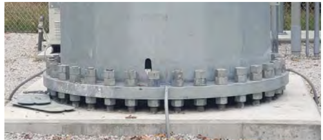
Locking nuts installed on all anchor bolts. Monopole has been grounded.
