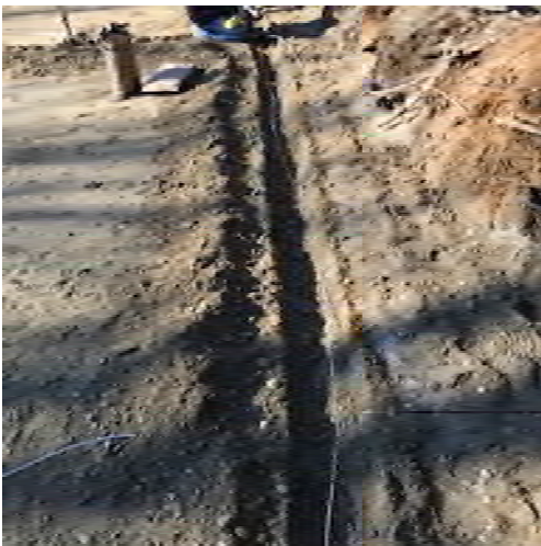
Ground ring installation (prior to backfill)
