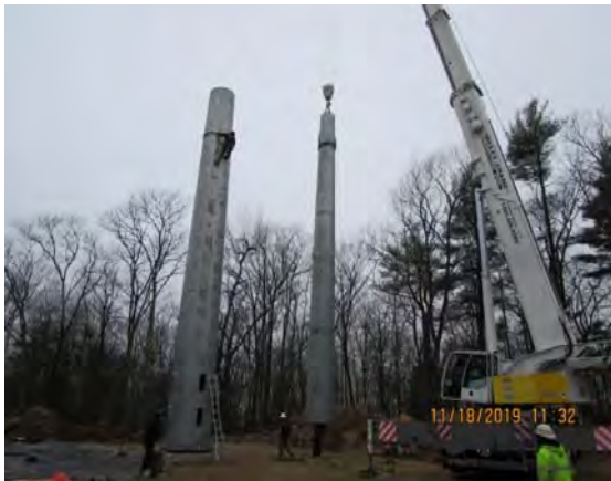
Stacking in progress
