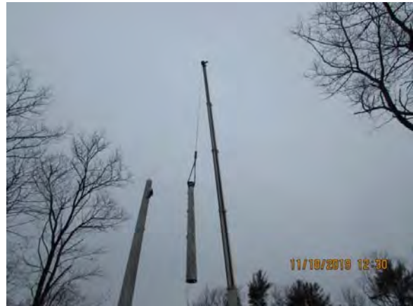
Tower stacking in progress
