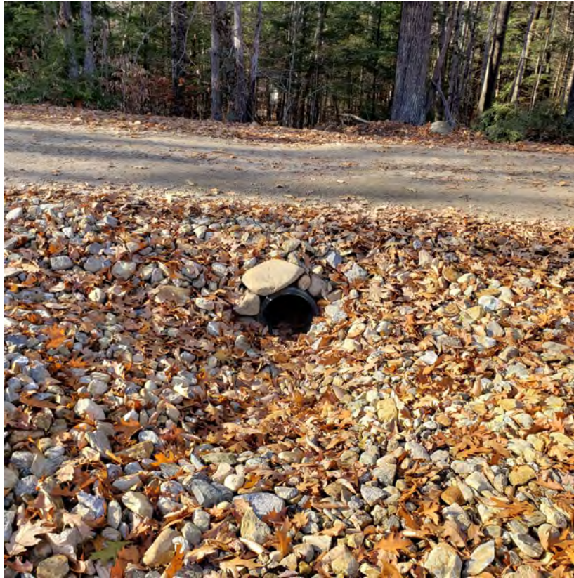
Bristol, NH – Driveway Culvert Outlet Protection
