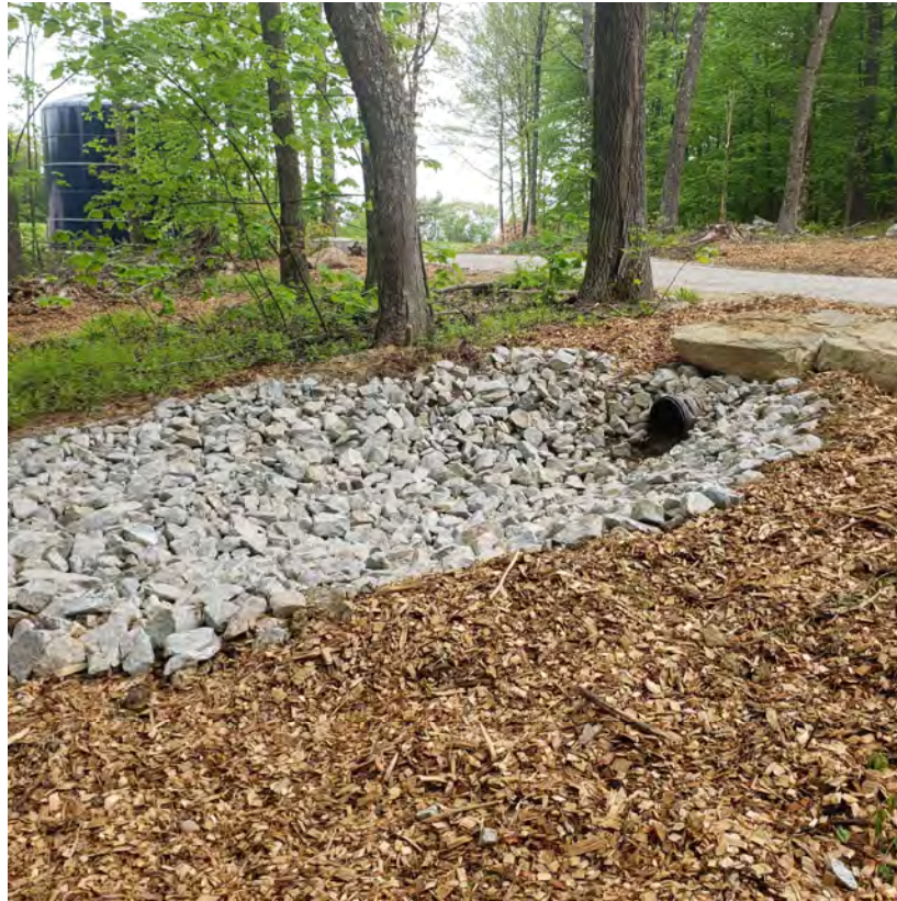
Monterey, MA – Culvert Outlet Protection and Woodchip Stabilization
