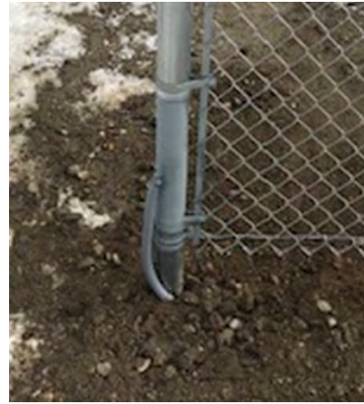
Typical fence grounding
