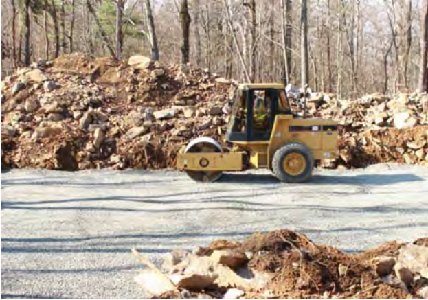
Tower foundation base compacted with a roller
