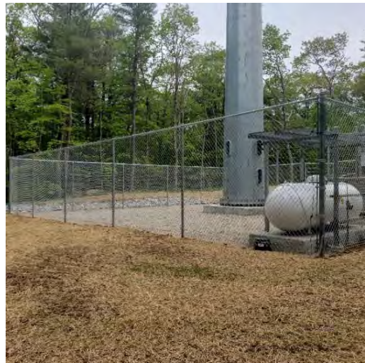
Chain link fence insrtalled
