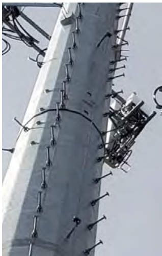
Safety climb installed (photo from a later inspection)
