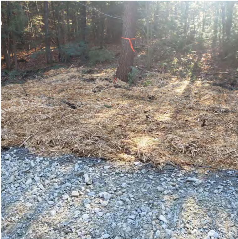
Henniker, NH – Wood Mulch Stabilization along Driveway
