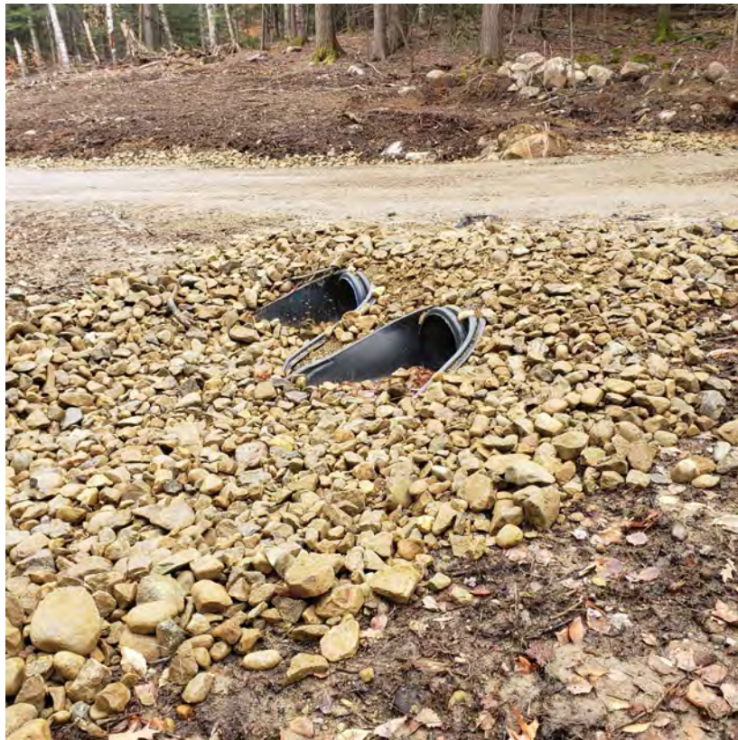
Bristol, NH – Driveway Culvert Outlet Protection
