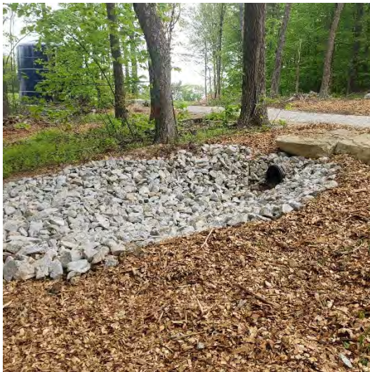
Culverts and stone headwalls
