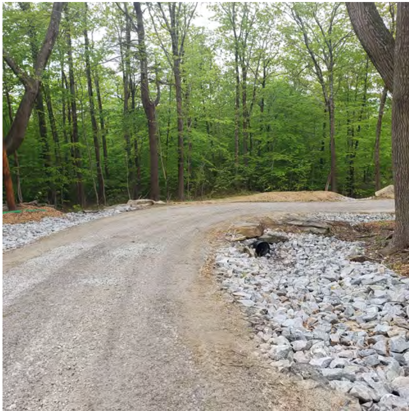
Monterey, MA – Culvert Inlet in Riprap Ditch
