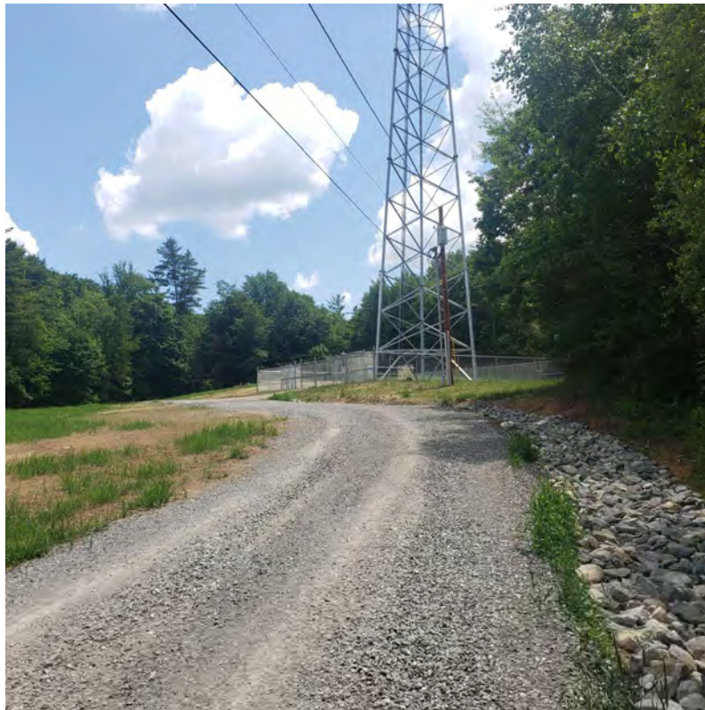
Bath, NH – Gravel Driveway with Riprap Ditch
