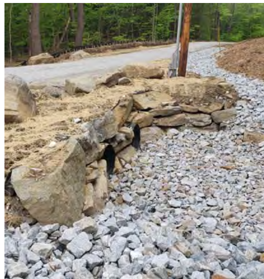
Culverts and stone headwalls
