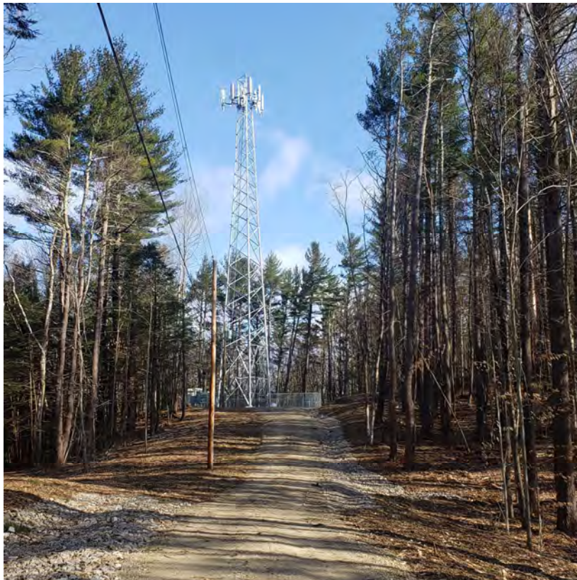
Colrain, MA – Driveway, Tower Compound, & Utility Run
