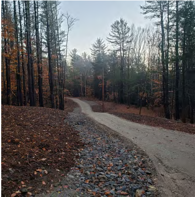
Colrain, MA – Gravel Driveway with Riprap Ditch
