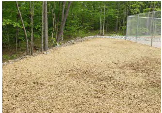
Disturbed areas seeded and hayed
