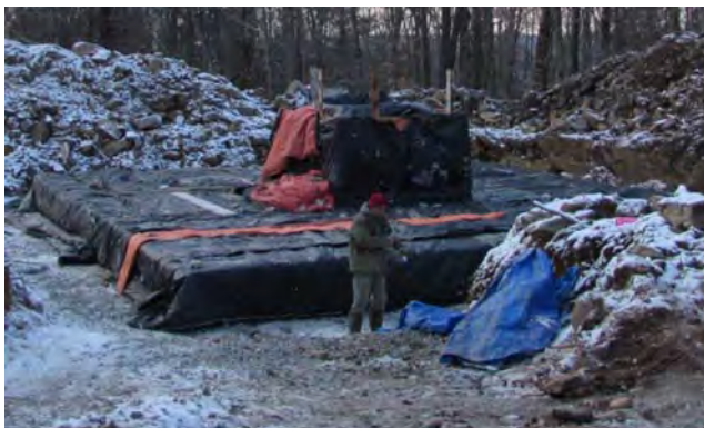
Concrete heat blankets on foundation
