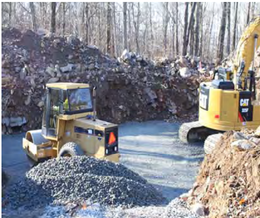
Foundation hole-post blast
