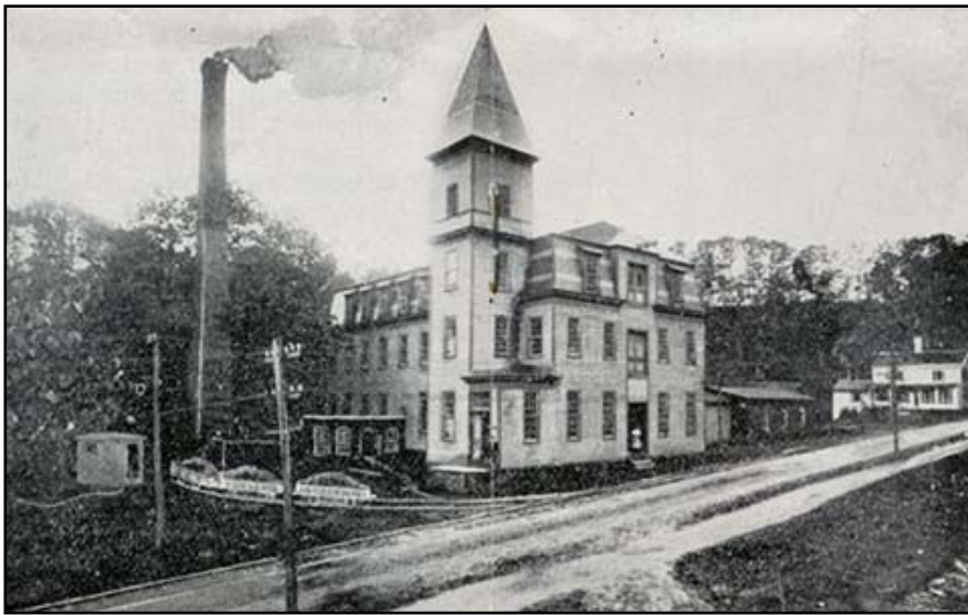
Tucker and Cook Upper Mill (photo from auction flyer, 1912, courtesy of the Conway Historical Society). This large cotton mill was fed by penstocks whose remains can be seen amidst the ruined mill foundation. Note trolley tracks and smokestack at boiler house.
