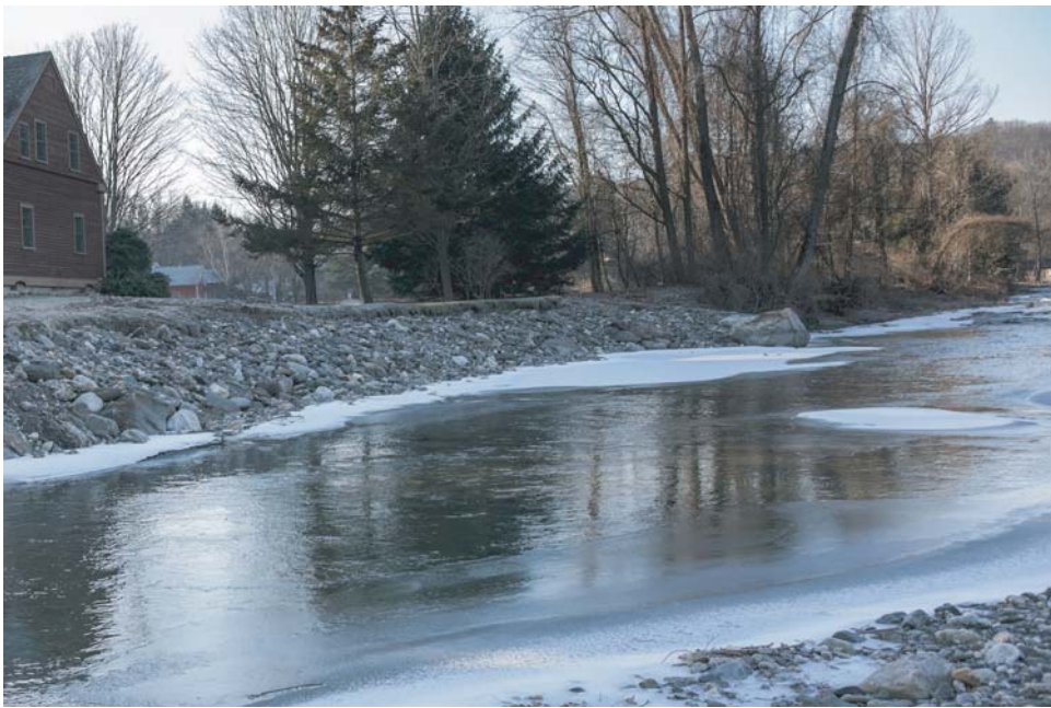
Emergency work - bank armoring following Tropical Storm Irene (courtesy of M. Turre)
