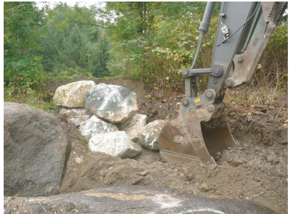
Constructing a boulder deflector
