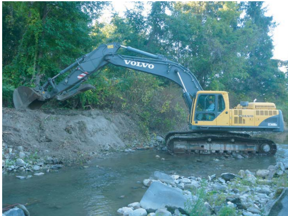
Excavation for deflector bank key
