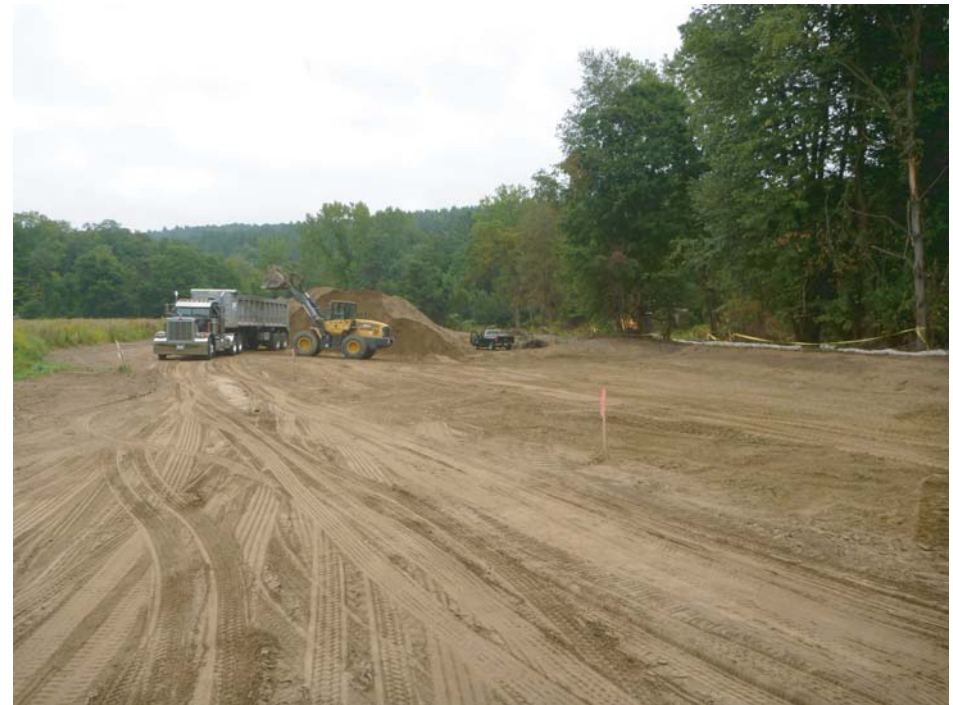
Floodplain lowering involved trucking loam off-site
