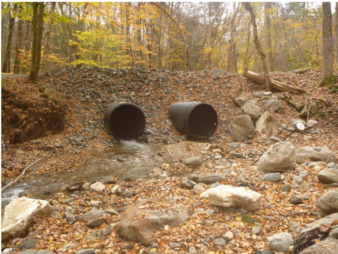
South River Walk and Watershed Tour - Stop 6. Adams Road crossing. The 7-foot diameter steel culvert washed out during the July 2023 floods and a) can be seen downstream; b) this has been replaced by two smaller culverts in the repaired road crossing.
