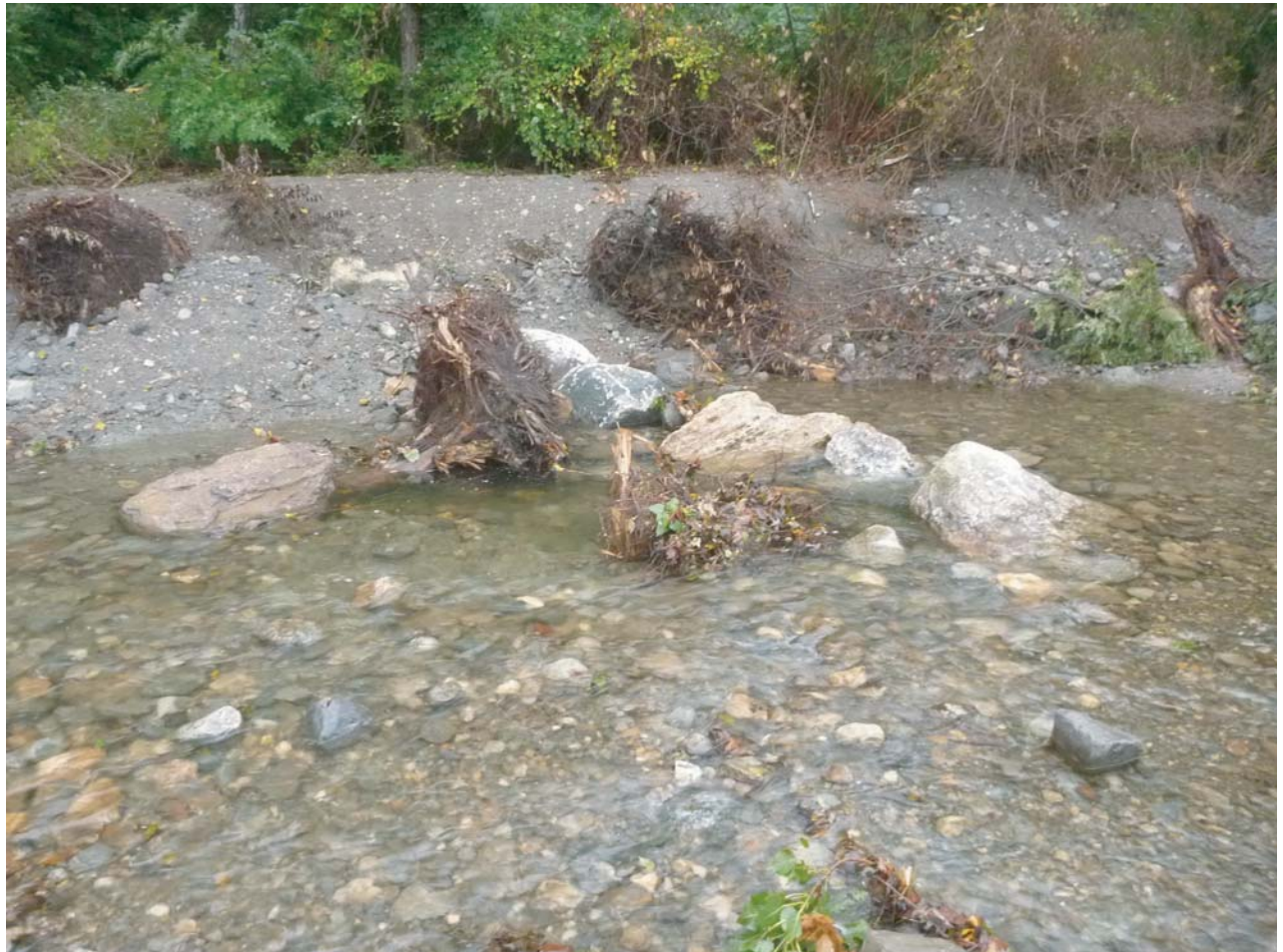
South River Walk and Watershed Tour - Stop 3. South River Meadow Site. Boulder deflector, just constructed on South River could be seen 2) turning water away from the bank at a flow of 60 cfs on September 19, 2016, and b) at base flow the next morning.
