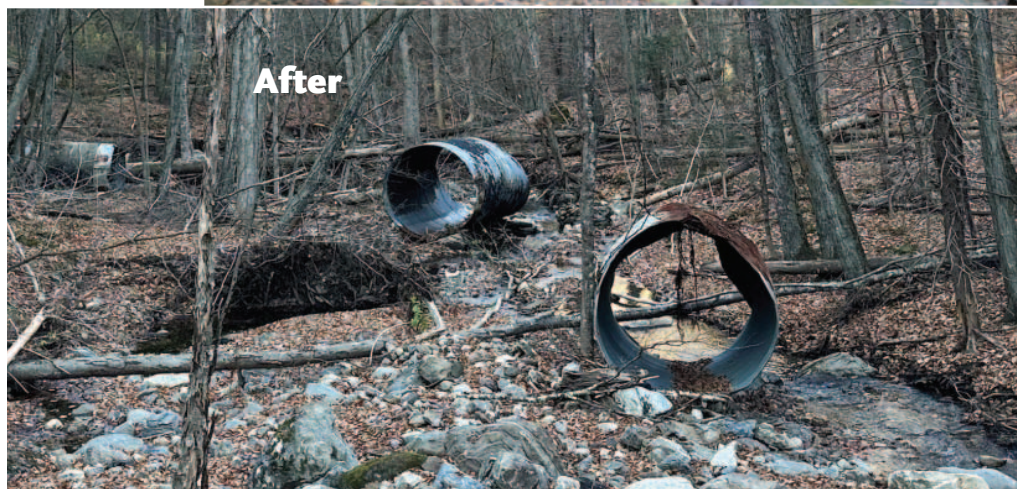
Top: Adams Road culvert, before the July 2023 storms. Bottom: Adams Road culvert washed out into three pieces, after the July 2023 storms.
