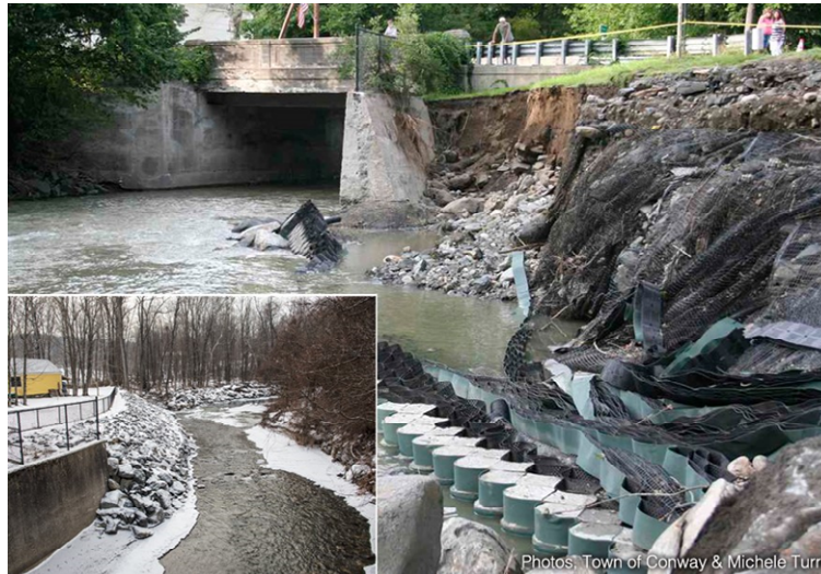
South River Bridge, Conway Center. Emergency Rip-Rap Repairs, 2011
