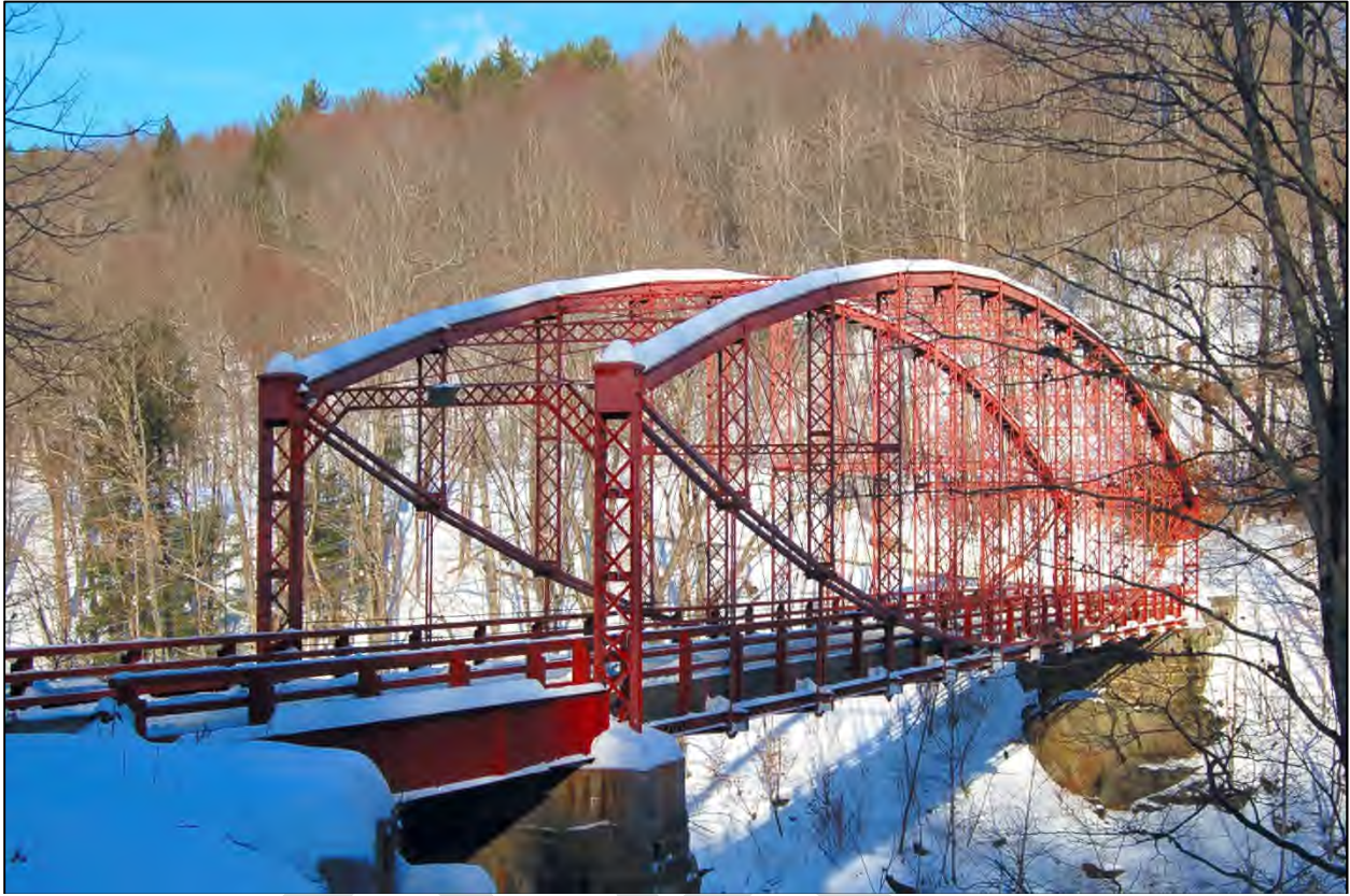
Bardwells Ferry Bridge ( David Chichester )
